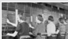
Operator Switching Stations
